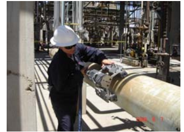
Vessel/Heater/Piping EMAT Services
