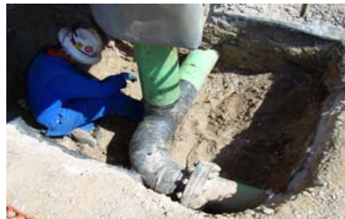
Soil to Air Corrosion Inspection
