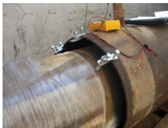
Cased Piping Inspection
